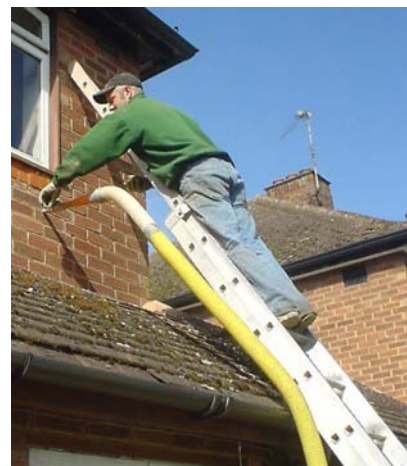
Figure 21.5. Cavity-wall insulation going in.
