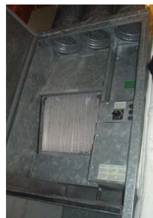
Figure E.11. The Heatkeeper's heat-exchanger.
