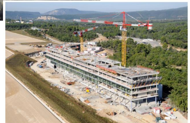
Facing the main entrance to the ITER site, the ITER Headquarters building will be the window to the ITER project for the world, Sept 2011.
